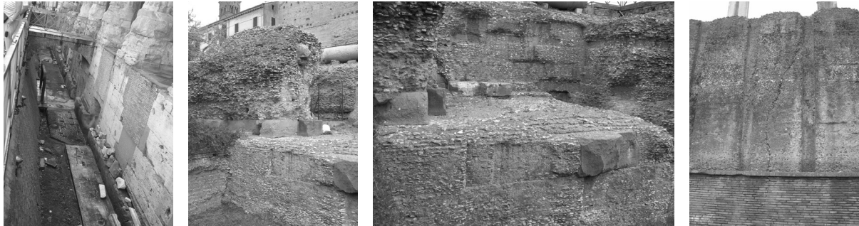
Figure 8: a) Foundations of the Temple of Hadrian b)-c) Voids left by the travertine and peperino foundations to the South of the platform d) Crack to the North side of the platform
