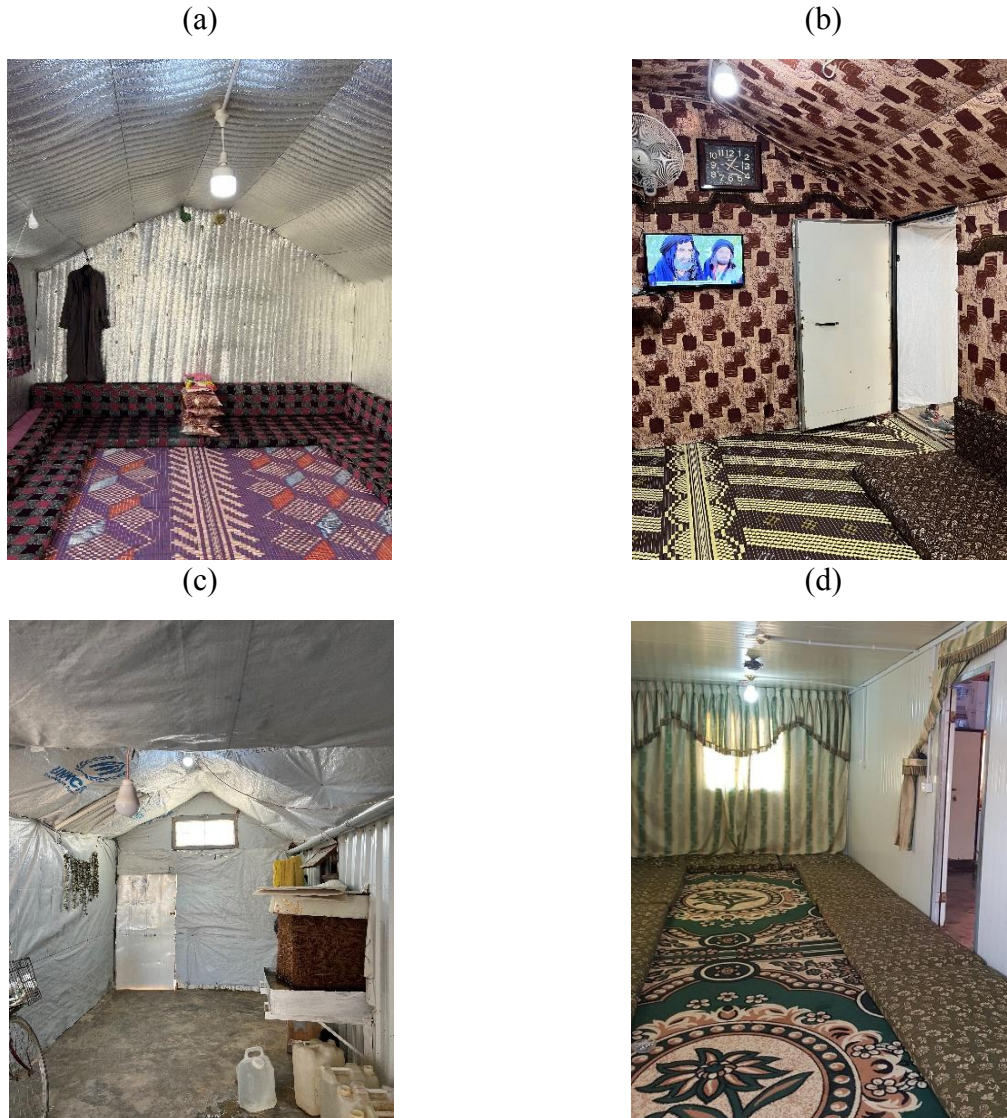
432 Figure 2: The interior of some shelters that could affect the development of fire: a) Foam lining and fuel loaded 433 furniture at Azraq camp- shelter 1 (Alshawawreh, 2022), b) Fabric lining and combustibile furniture at Azraq camp- 434 shelter 3 (Alshawawreh, 2022), c) Plastic lining at Azraq camp- shelter 3 (Alshawawreh, 2022), d) A shelter's 435 interior at Zaatari camp- shelter 4 (Alshawawreh, 2021)
