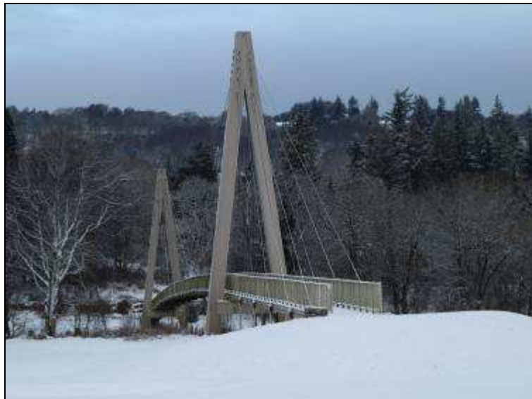
Figure 1. Aberfeldy footbridge from the south (December 2010).
