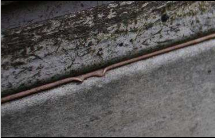
(a) GFRP and adhesive joint condition on bridge deck
