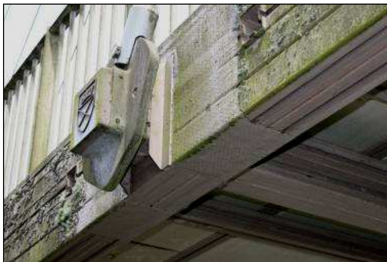
Figure 6. CFRP strengthening retrofitted around a primary transverse beam (June 2008)
