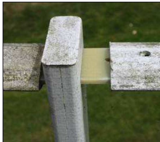
Figure 12. Details of the connection between the top handrail and parapet post (June 2008).
