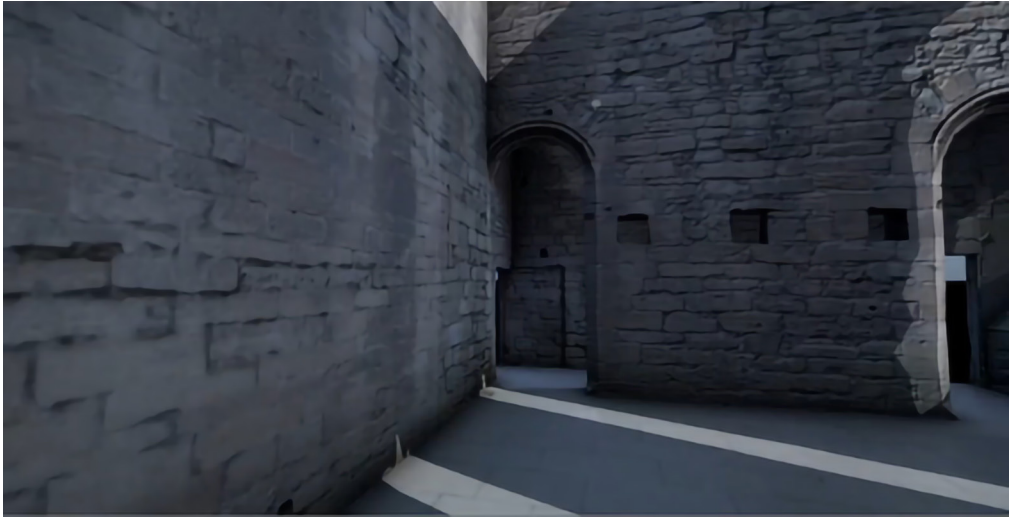
Figure 3. Linlithgow palace chapel as it stands today, reconstructed from LIDAR scanning with overlaid textures
