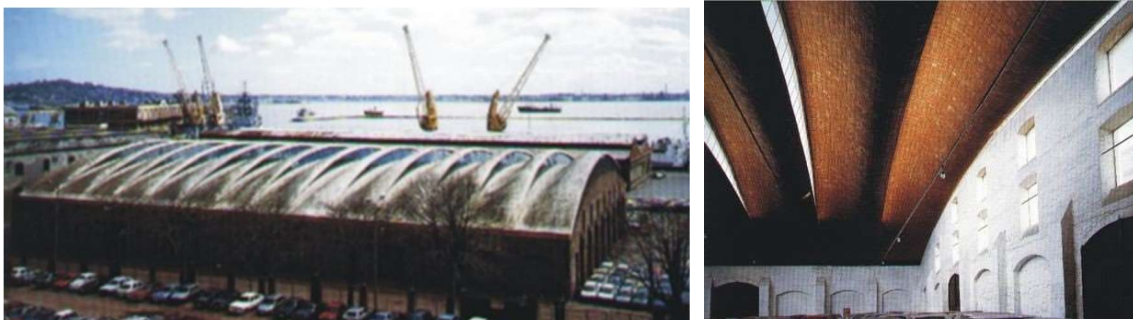
Figure 3. Julio Herrera y Obes Warehouse, showing use of vault for lighting
