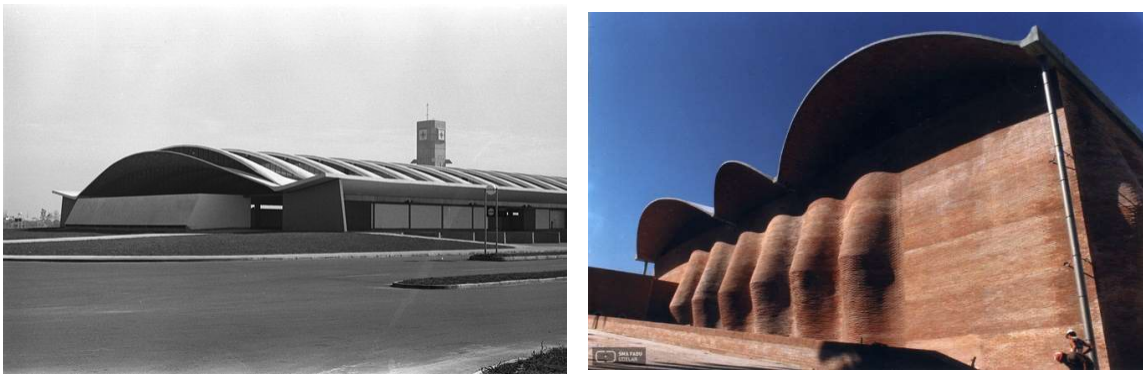
Figure 4. Citrus Caputo, showing the edge condition and Montevideo Shopping showing the combination on Barrel and Gaussian Vaults
