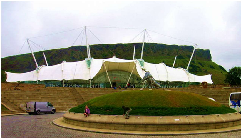
Figure 2 Dynamic Earth Building at the foot of Salisbury Crags in Edinburgh
