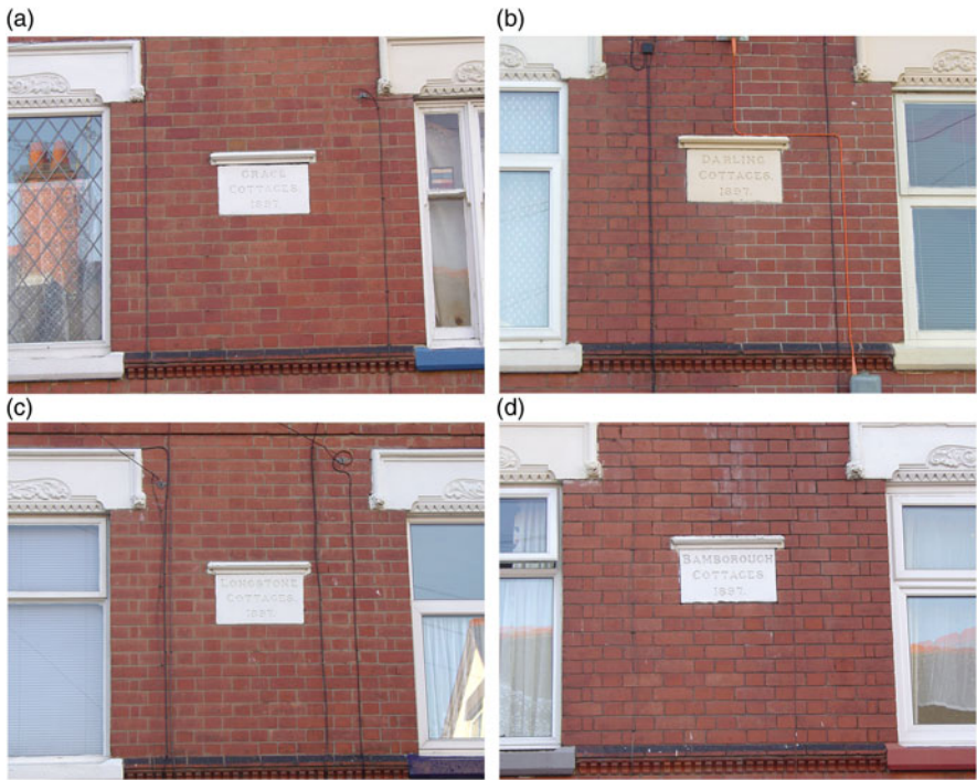
Figure 6a-d. Historical events recorded on house facades: shipwreck 1838. (a) Grace (b) Darling (c) Longstone (d) Bamborough; 26-38 Tyrell Street.
