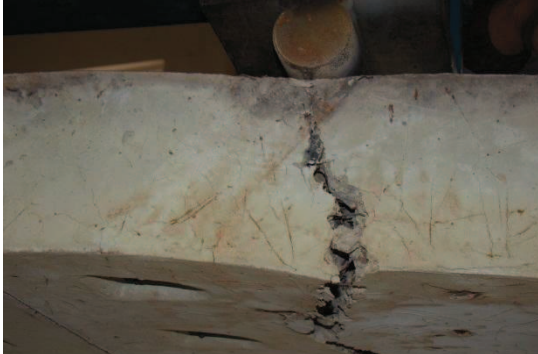
(h) Concrete fracture (HFRCJ4)
