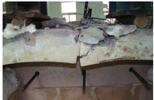
(g) Joint concrete failure (RCJ4)
