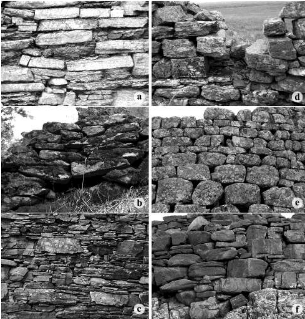
Illus. 6 Masonry patterns built of locally available stone material: a) sandstone: Hillock of Burroughston, Shapinsay, Orkney Islands; b) schist: Druim An Duin, North Knapdale, Argyll and Bute; c) gneiss: Dun Troddan, Glenelg, Highland; d) gneiss: Dun Borge, Barvas, Lewis, Western Isles; e) basalt: Dun Hallin, Duirinish, Skye, Highland; f) sandstone: Clachtoll, Assynt, Sutherland, Highland (Photographs: T. Romankiewicz)
