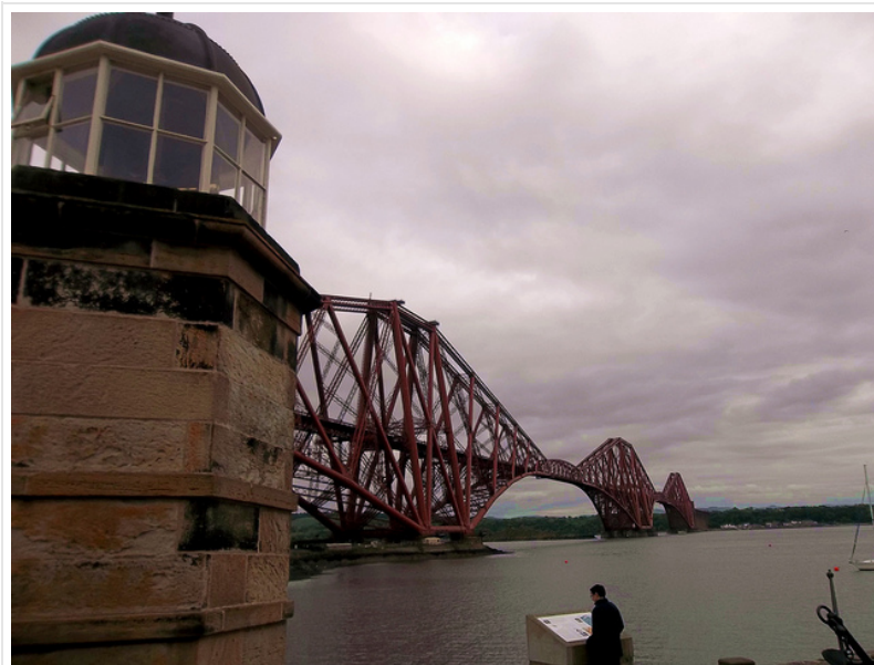
The Bridge to Independence? (Andrum 99, CC BY 2.0)
