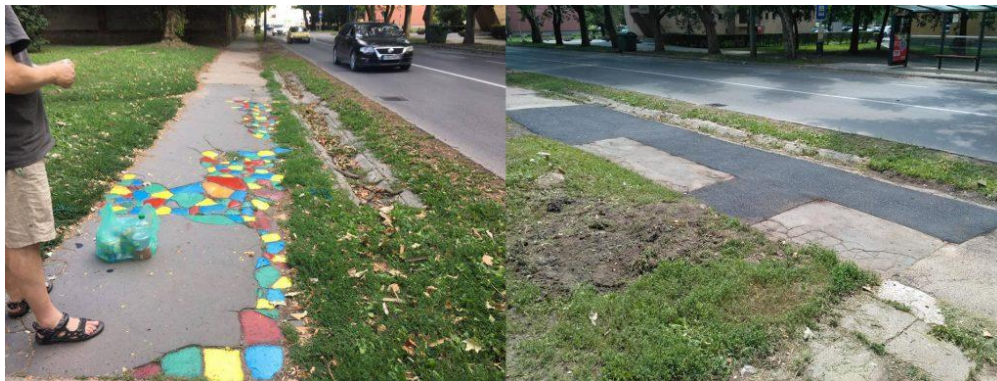
Figure 7: Repaired sidewalk following an MKKP intervention 4
