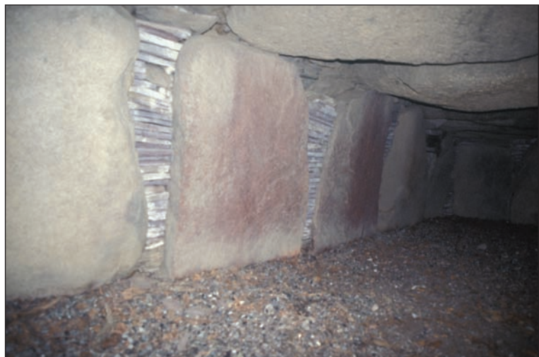
Fig. 3. Orthostats and dry-stone walling at the passage grave of Knudshoved, Zealand.
