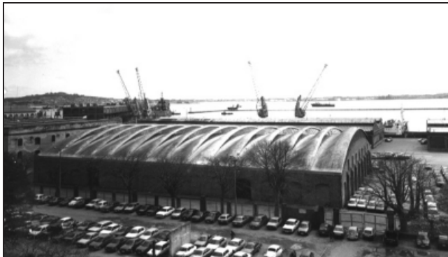
Fig. 13. The JHO warehouse at Montevideo Docks (Dieste Archive)
