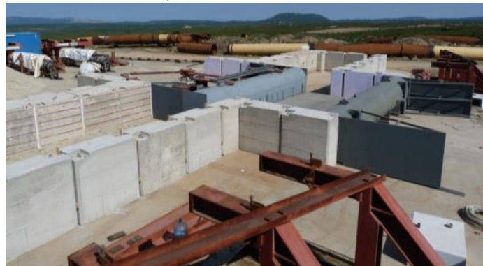
Figure 28. Soil boxes before sand filling and pipe specimen installation.
