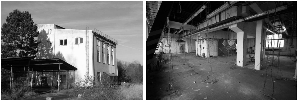
Figure 5: Left – Southwest corner of test building, and Right – fire compartment
