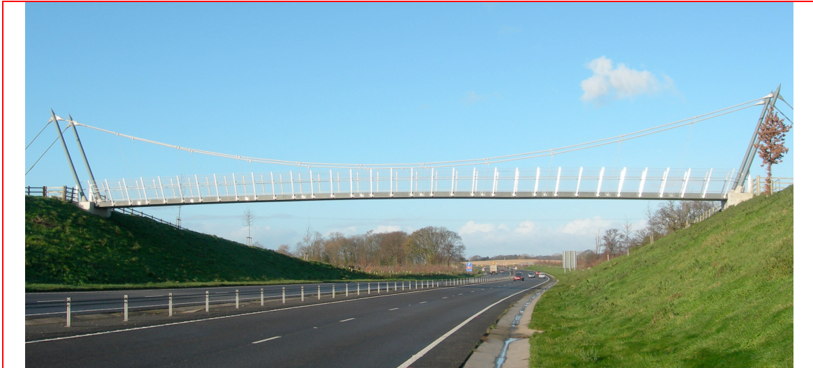
Fig. 1 An overview of the completed Wilcott footbridge.
