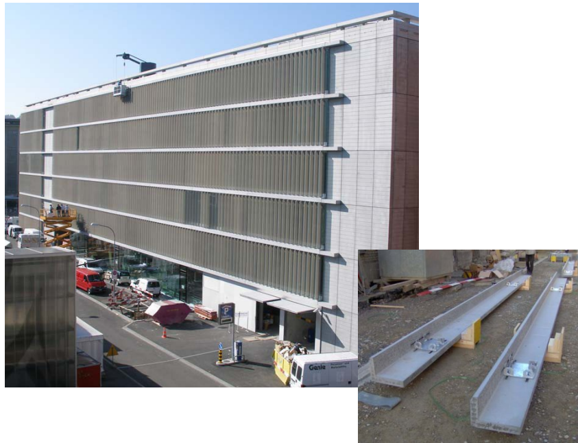
28 Figure 1 – Application of CFRP prestressed concrete L-shaped beams for structural façade elements in 29 Zurich, Switzerland [1].
