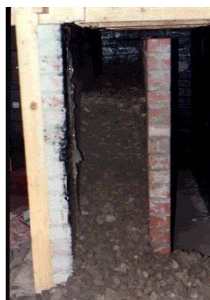
Figure 3 Tank containing 0.75m of spent ballast (Clark M. , 2001)
