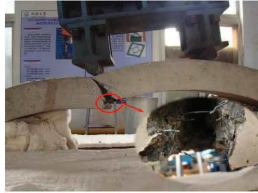
(b) Steel fiber failure under thermal-mechanical loading
