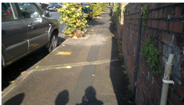
Figure 2. Changes in levels – drain across pavement
