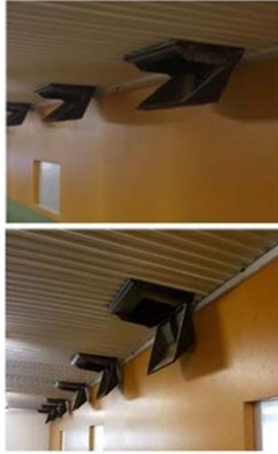
Figure 2: Schematic description of the operation of the 'increased air velocity at pig lying area' pig-cooling strategy. The top figure illustrates air distribution with a maximum 75% air inlet opening, while the bottom figure illustrates air distribution with fully open (100%) air inlets. Irregular lines depict the slatted, excretory area of the pen.
