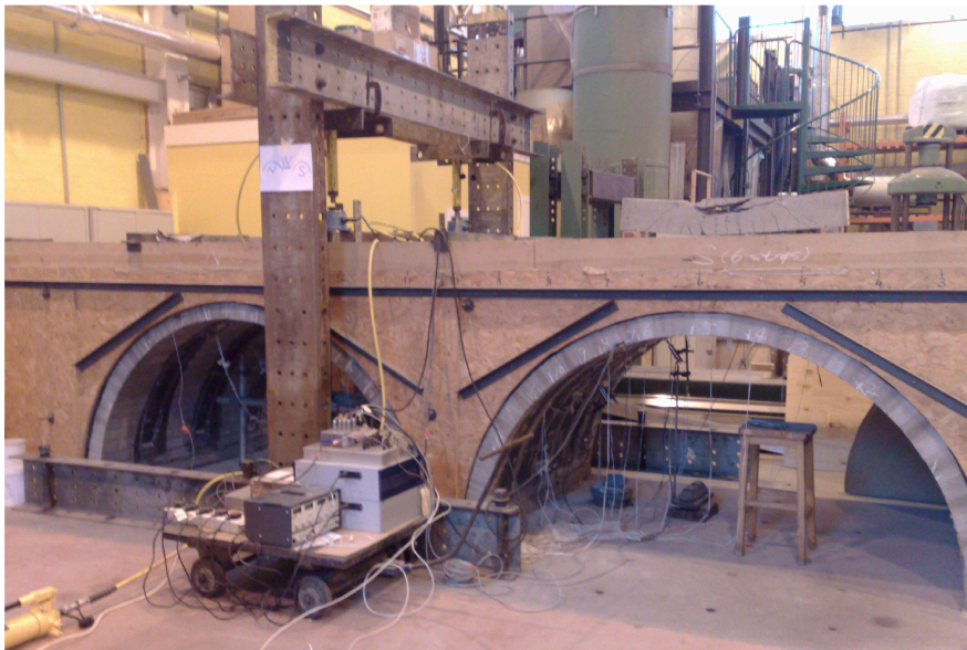
(b) Photograph, taken from the west side after strengthening
