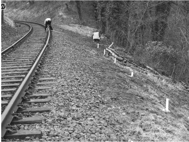
Figure 5. Setting out telltales in a priority area
