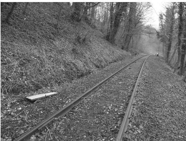
Figure 2. The Bo'ness and Kinneil Railway, showing typical cutting and embankment structure
